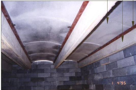
INTERIOR VIEW OF THE FINISHED JOIST AND PAN CAST IN SITU
